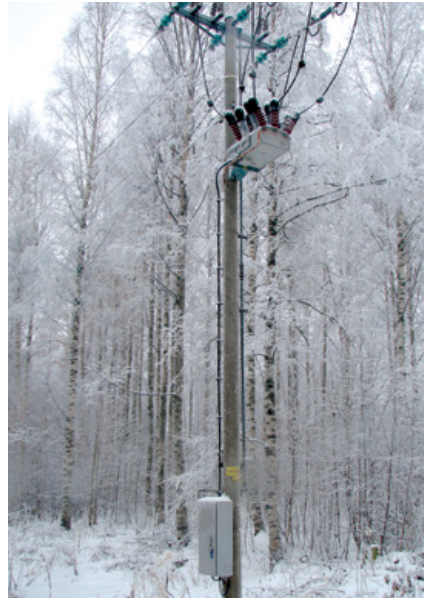
OSM RECLOSER AND CONTROL AND COMMUNICATIONS CUBICLE
